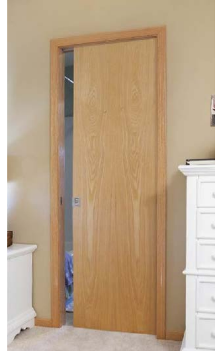
POCKET FRAME COMPONENT INSTALLED
